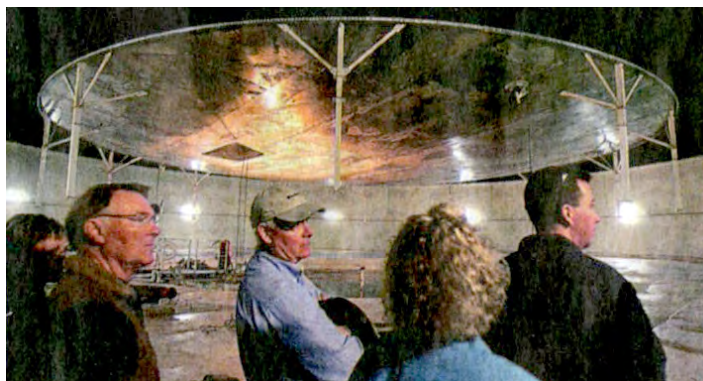
"The Lung" regulated air pressure and flow into the facility in the years when eight people — the Biospherians — went inside to use it as a model for moon and Mars bases.
